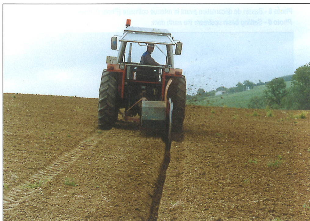
Photo 4 - Drain-laying across the slope.
